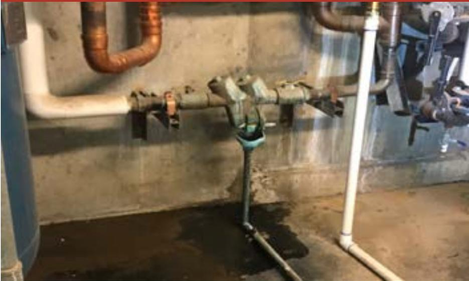
Old Pressure Relief Valve (PRV) that has rusted out over the years and leaked badly.
